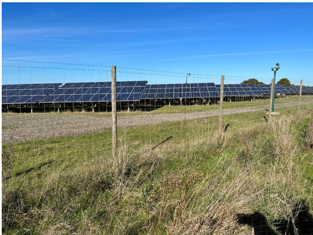
Plate 4: Example of mesh stockproof fencing and a metal perimeter CCTV pole
