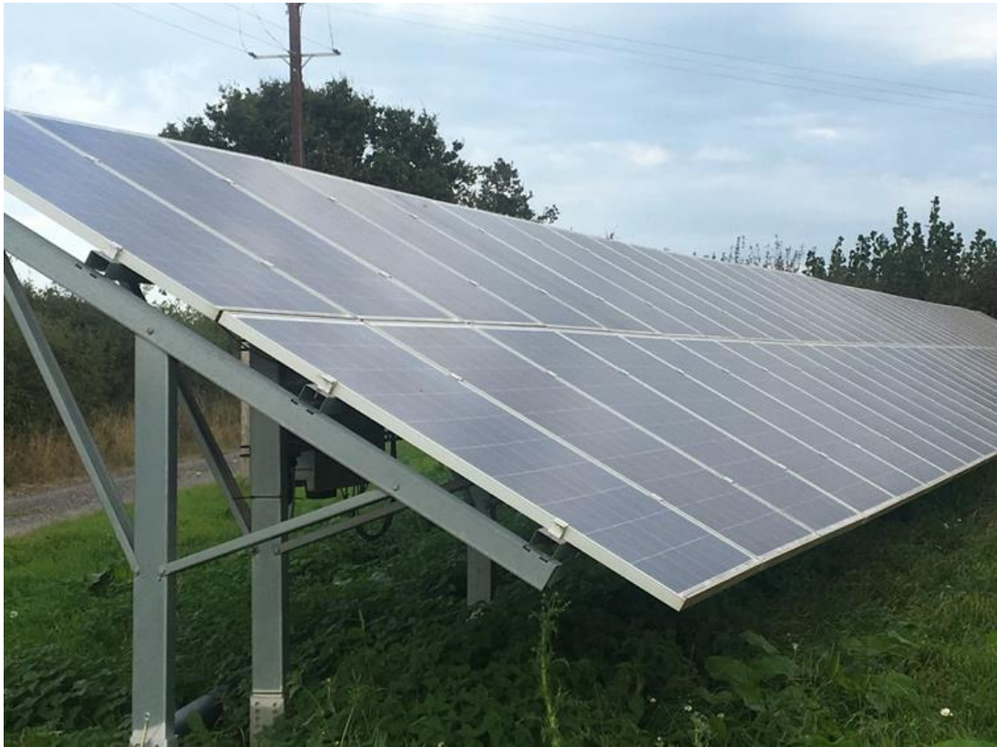
Plate 1: Solar PV Panels with Fixed South Facing Configuration
